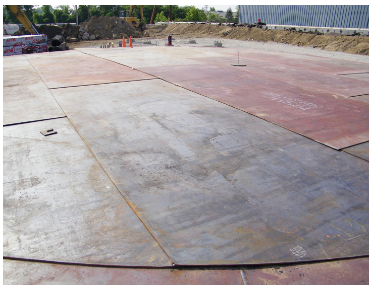
Figure 1. New tank bottom installation.
